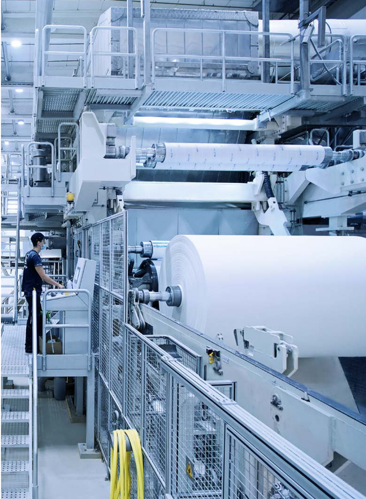
The ANDRITZ tissue production plant at Vajda Papír in Hungary was started up with the help of the Metris Performance Center and is an example of how resource-saving components can be combined with advanced automation solutions.
