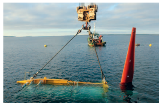
Installation of HS1000 at EMEC
