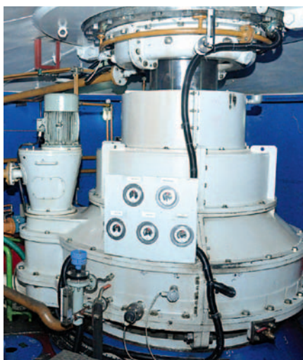
Turbine pit after renovation
