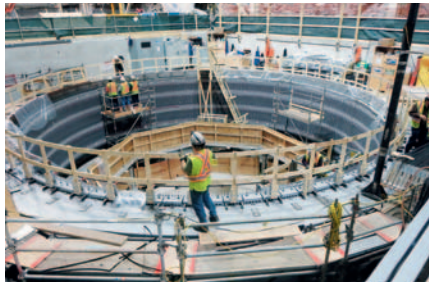
□ Stator assembly
