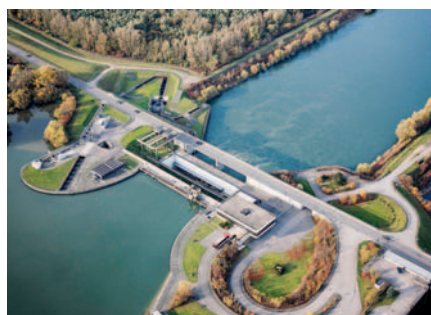
□ Bird's eye view of the hydropower plant
