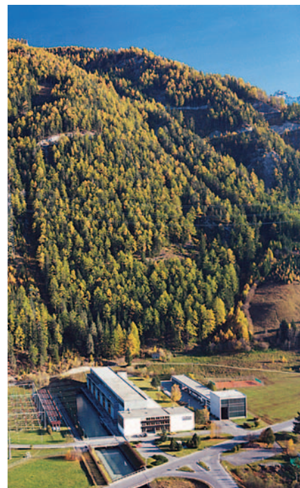
▣ Power house and switchyard
