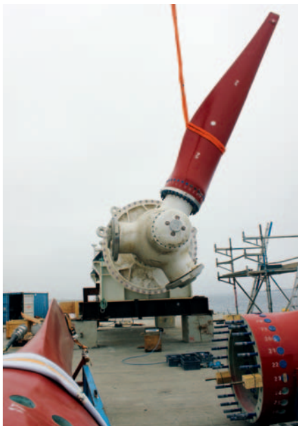
Installation of HS1000 at EMEC, Scotland
