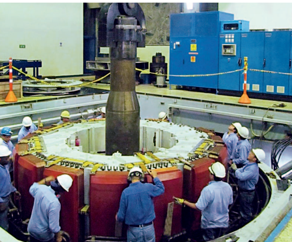
□ Rotor installation
